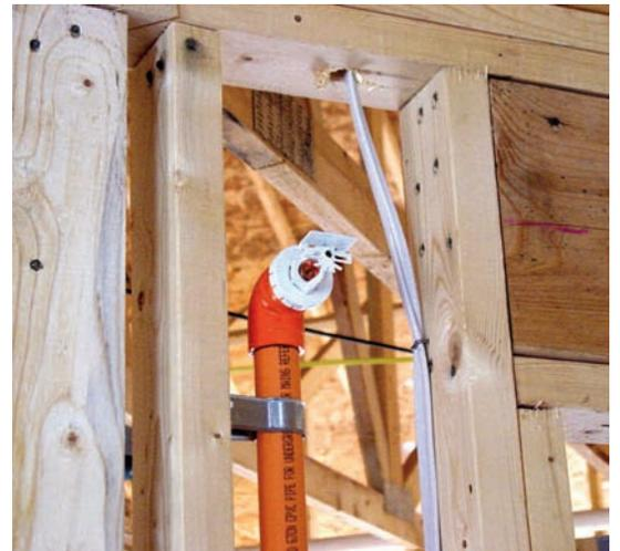
**Photo 17: Residential sprinklers installed during construction. Much of the system may be installed using plastic pipe.**
