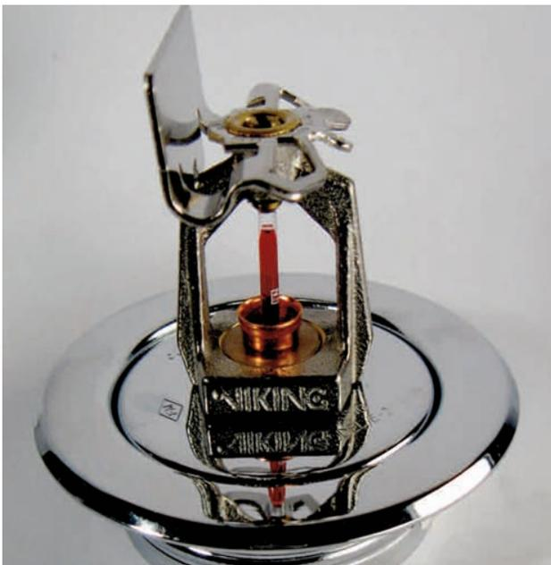
*Photo 15: 2003 Viking Model E-2 Sidewall Quick-Response head for residential use.*
