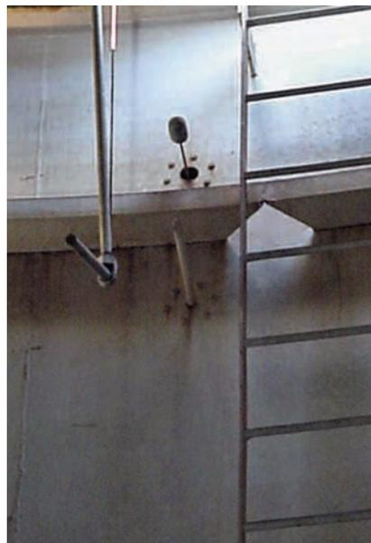
*Low water level alarm device and low water temperature alarm devices located near the top of a steel suction tank. The ladder leads to the roof access port.*
