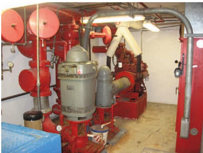
*The floor of this fire pump room also serves as the top of the below-grade concrete tank. Two vertical turbine fire pumps are extended into the tank to supply protection water for the sprinkler systems. The pump in the foreground is driven by a vertically mounted electric motor. The pump in the background is driven by a horizontal diesel engine with a right angle drive on the top of the pump.*
