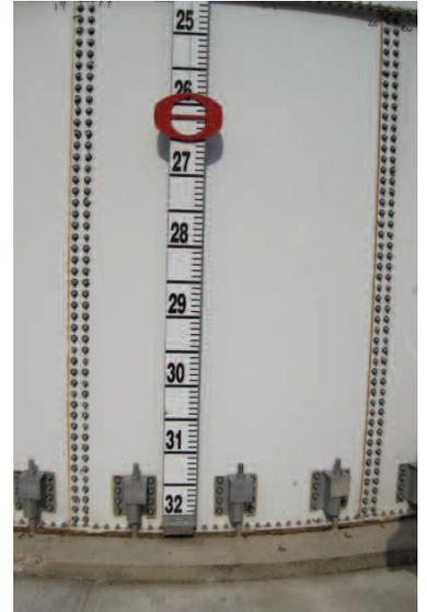
*This is a ground-level suction tank supplying a fire pump. Note the construction of this tank is steel, which has been bolted together. This tank is located in an earthquake-prone area, and foundation bolts have been installed around the tank base to help hold it in place during an earthquake. The tank water level indicator shows that the tank level is at approximately 26 ft of the 32 ft of tank height.*
