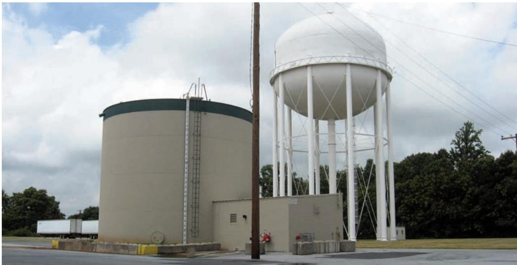
Many industrial facilities rely on elevated gravity tanks plus suction tanks and fire pumps for adequate fire protection water supply.
