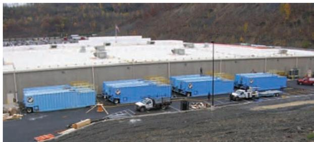
*During an impairment of the water supply to this facility, portable tanks were delivered to the site and connected to the fire pump. Fire protection was maintained in service due to proper impairment handling procedures.*
