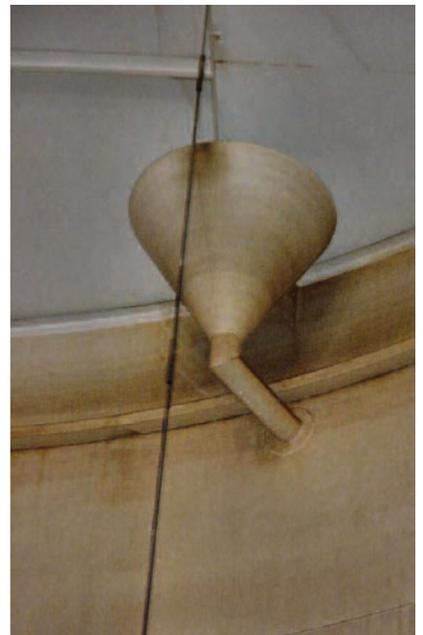
*The overflow of a tank is typically a funnel attached to a pipe, which extends through the tank wall. This is a welded-steel, ground-level suction tank.*
