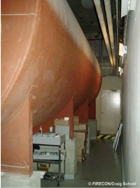
*A steel tank installed in the penthouse of a high-rise building as a gravity tank. Concrete tanks may also be used as a gravity tank.*
