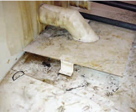
*This is a vortex plate inside of the fire pump suction tank. It prevents a vortex (a swirling funnel, which allows air into the suction pipe and fire pump). The anti-vortex plate is required equipment in a suction tank. This is a welded steel tank. The floor is constructed of steel panels laid on fill material. Setting of the fill material can create voids under this steel floor.*
