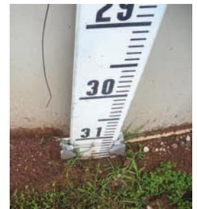
*The tank water level indicator is not functioning because the cable to the float inside of the tank has become disconnected. The indicator has dropped to the ground. This is a welded steel tank.*
