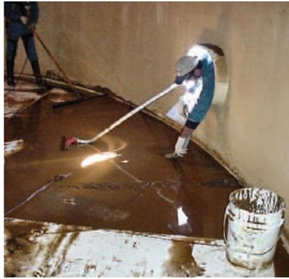
*Over time, a significant amount of silt and sediment accumulates inside a tank. This material should be removed when internal tank maintenance is performed.*
