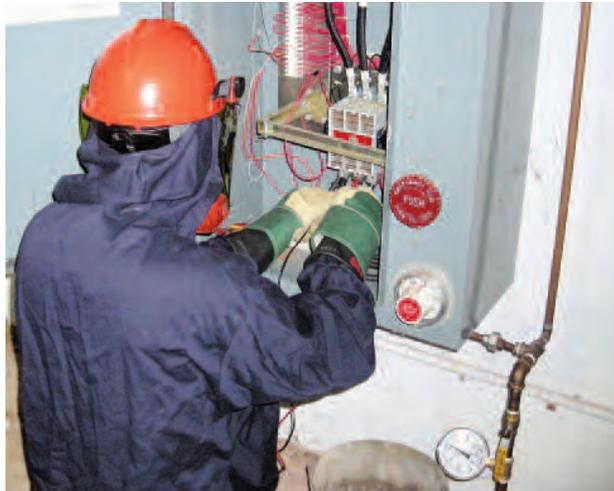
*Photo 10: Technician taking voltage readings during a fire pump test. The emergency run knob is at the lower right of the control panel. Pushing this knob and locking it in place will engage the contactor to start the motor.*
