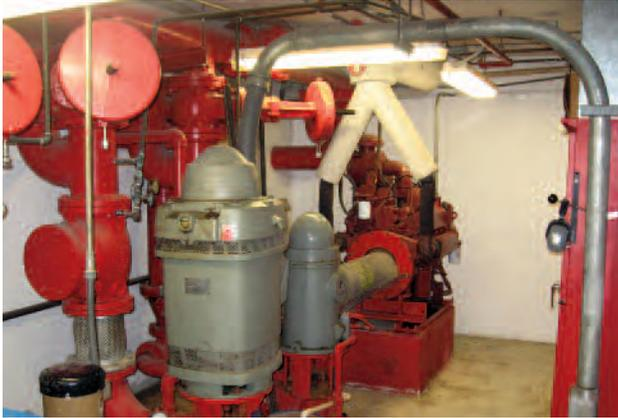
*Photo 5: Two vertical turbine fire pumps taking suction from a reservoir. The pump room floor is the top of the water reservoir. The near unit has an electric motor mounted vertically on the pump. Behind is a diesel driven vertical turbine pump with a right-angle drive.*
