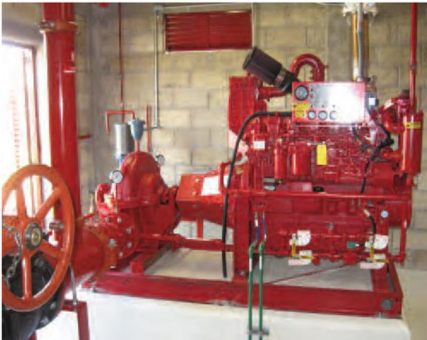
*Photo 6: A diesel-driven horizontal split-case fire pump. The instrument panel is at the top of the engine. The cooling line and bypass are located alongside of the engine. The batteries are located on the opposite side of the engine so the operator does not stand in front of, or reach over them, to operate the pump.*
