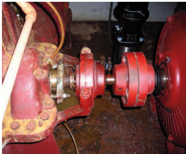
**Photo 4:** The packing glands are located where the shaft enters the pump. The inboard bearing is on the pump housing frame. The flexible coupling is located between the pump and the driver.
