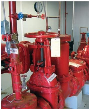
Fire pumps supply adequate pressure and volume for many fire suppression systems. In this impairment, the pump's main discharge valve is shut off.
