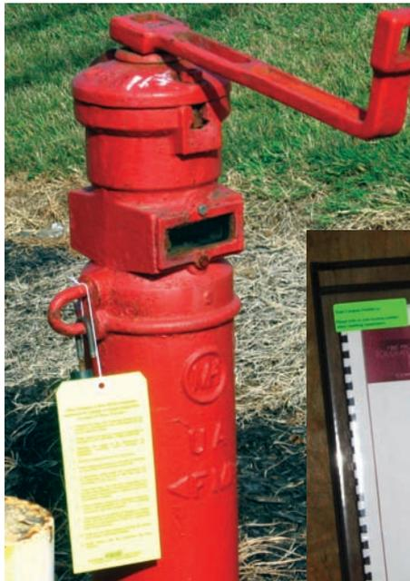
(Left): This post indicator valve is shut off and has been tagged as impaired.
